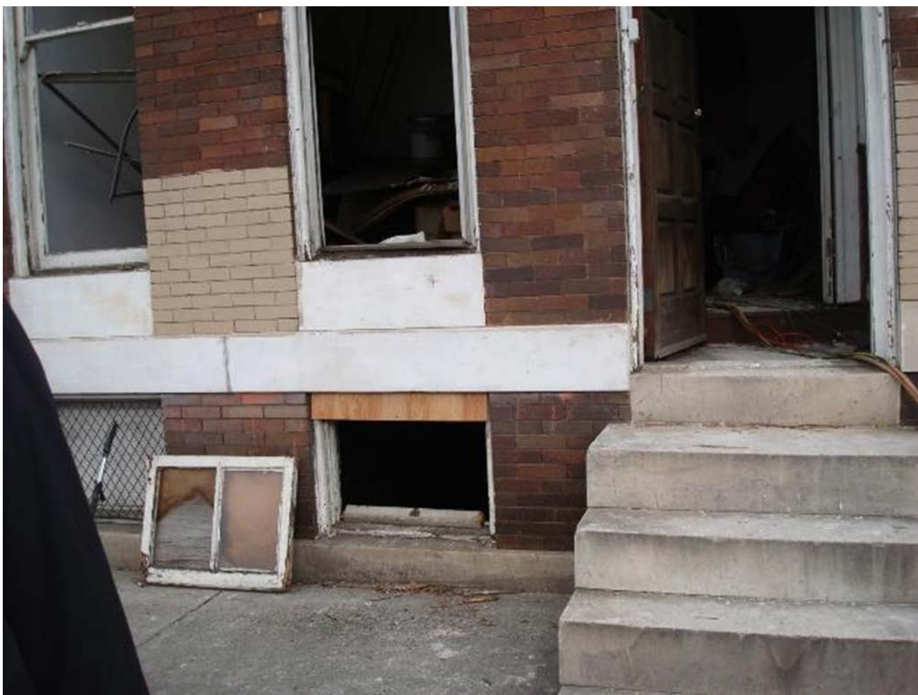
Photo 8. Photo shows basement window at Side Alpha of the Delta exposure building removed as part of the NIST data collection process. This window was not opened the night of the incident. (Photo NIOSH)
