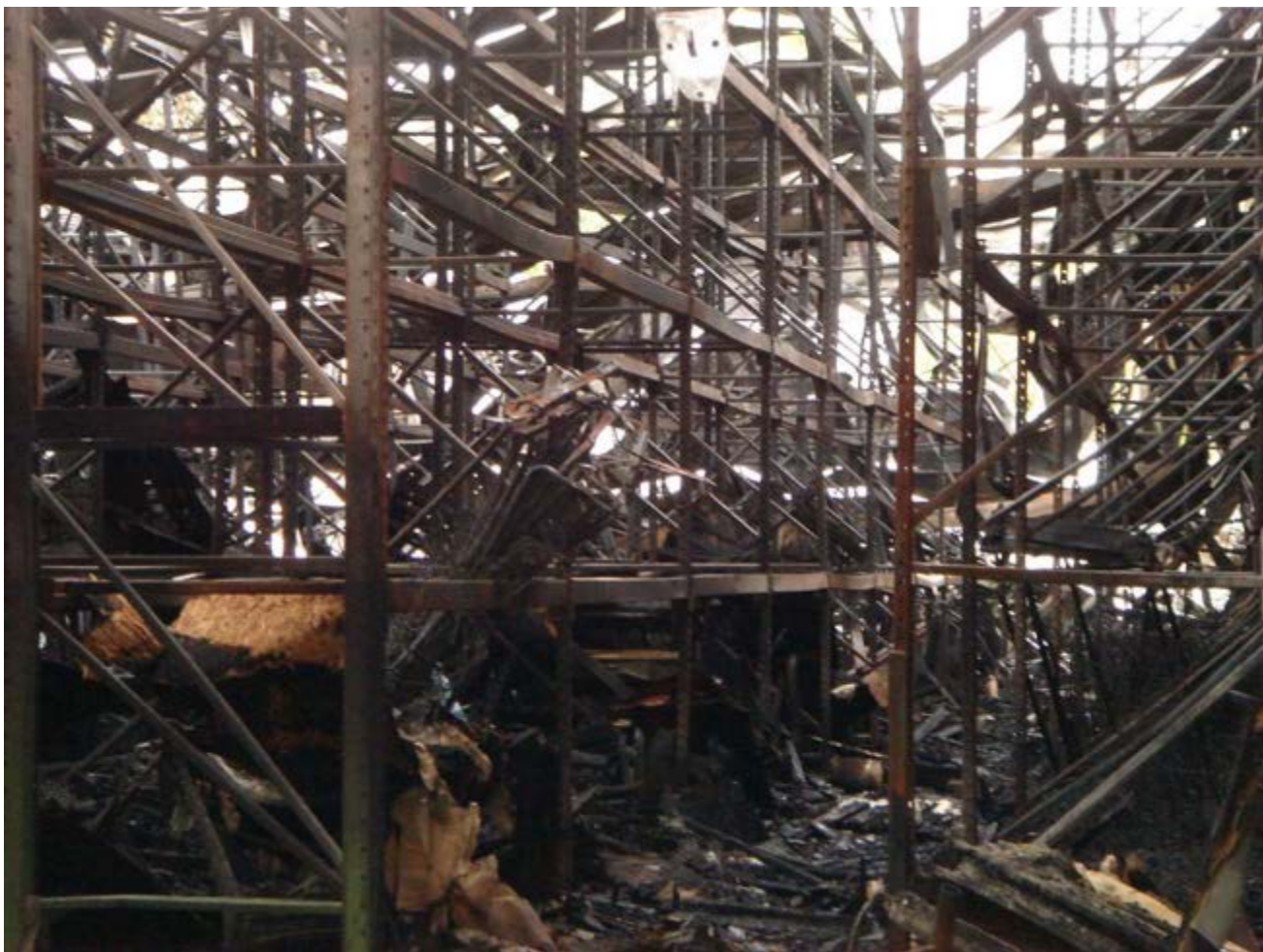
Photo 9. Storage racks in warehouse post fire. Storage racks were filled with various furniture and mattress items. Note the extent to which the storage racks filled the warehouse which gives an indication of the volume of merchandise and the fuel load inside the 15,600 square foot warehouse. The warehouse measured approximately 130 ft. by 120 ft. and was 29 ft from floor to roof. (Photo – NIOSH.)
