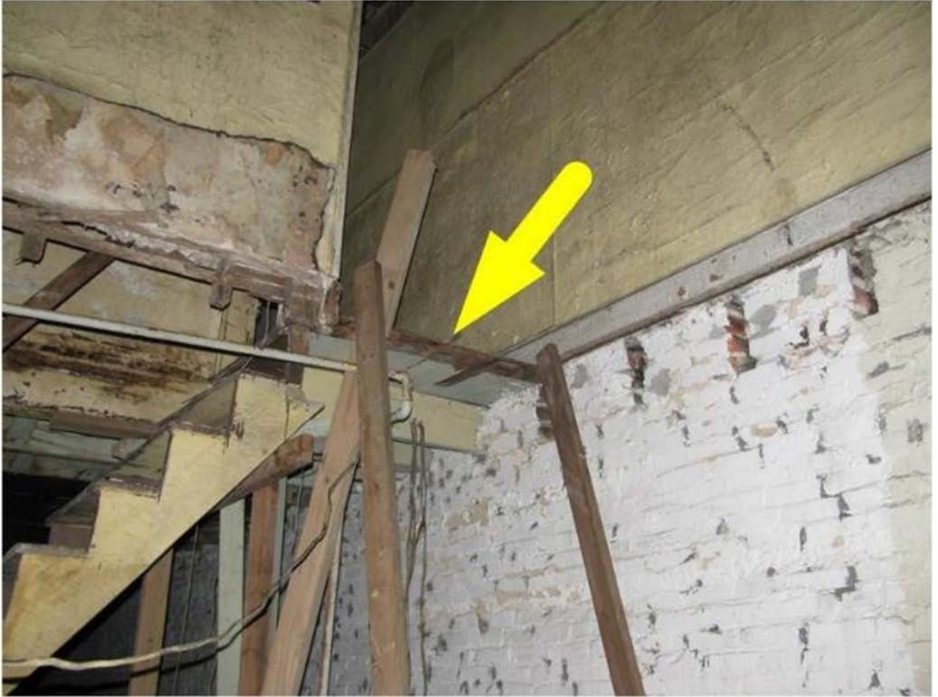
Photo 4. View of the missing floor taken from near the approximate location where the shift safety officer likely landed on the basement floor. It is believed he stepped off the first floor at the area highlighted by the arrow.
