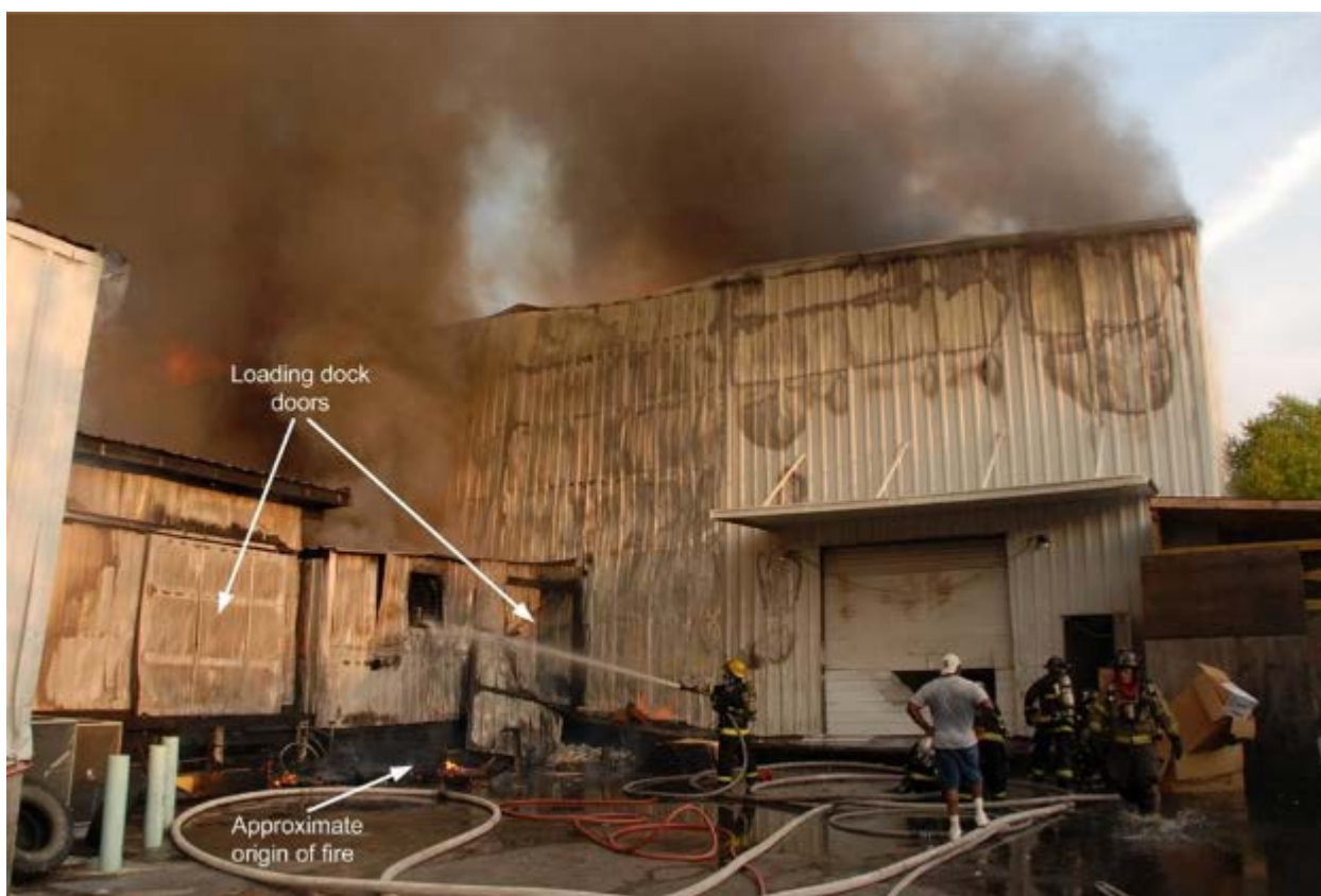
Photo A-2. Time is approximately 1936 hours. Loading dock area approximately 20 minutes after first crews arrived on scene. There is heat damage to metal siding on loading dock and warehouse. There are two Loading dock doors. There is an approximate origin of fire in the corner. (Photo courtesy of Police Department, Bill Murton, photographer.)
