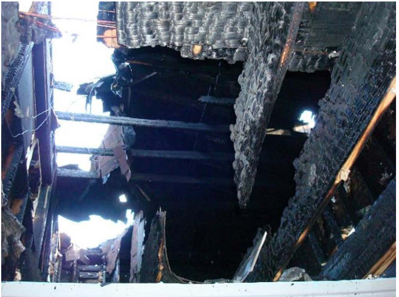
Photo 4. Large void space over the garage at the Alpha/Delta corner connecting the L-shaped attic structure. (NIOSH photo.)
